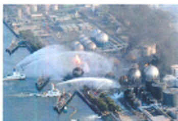
Fukushima nuclear plant post-earthquake, Japan
